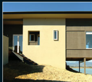
House on Waimea Inlet Irving Smith Jack Architects Ltd
