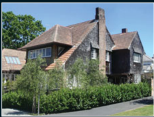
Paterson House Robin O'Donnell Architects Ltd
