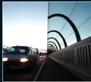
Grafton Bridge Safety Screens GHD Limited
